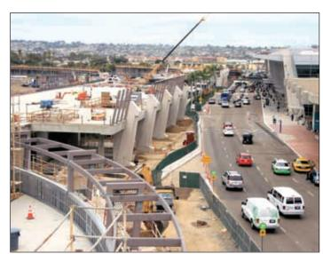
Lindbergh Field has reached the halfway point of its \$1 billion Green Build that will include 10 new gates, a new flight tower, "smart curbs," an expanded concession areas and, shown here, an elevated departure roadway next to a new United Services Organization (USO) building Photo by Don Balch I The Beacon
